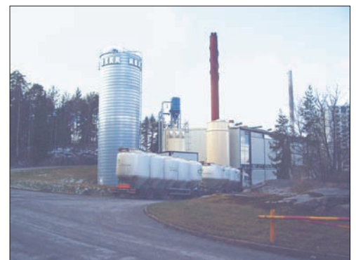
Loading wood pellets.
