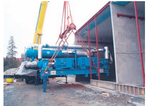
The first unit being installed
