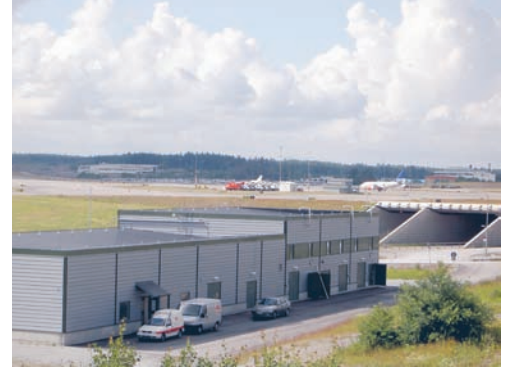
The district cooling plant is 1.5 km away from the terminal buildings.
